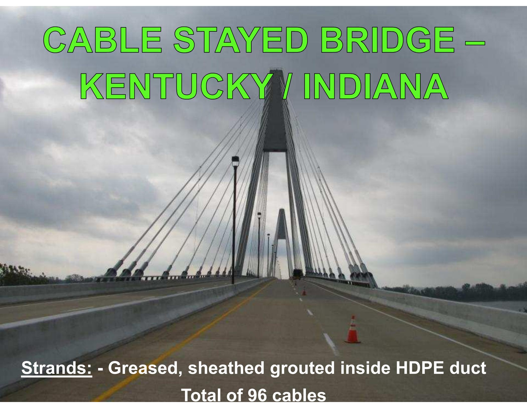
Strands: - Greased, sheathed grouted inside HDPE duct
